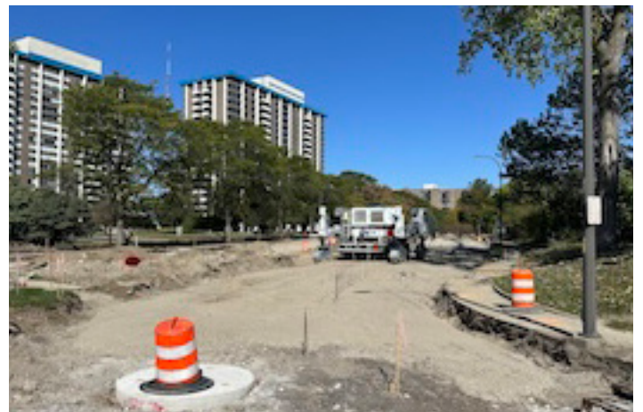
North Park Drive undergoes complete replacement
