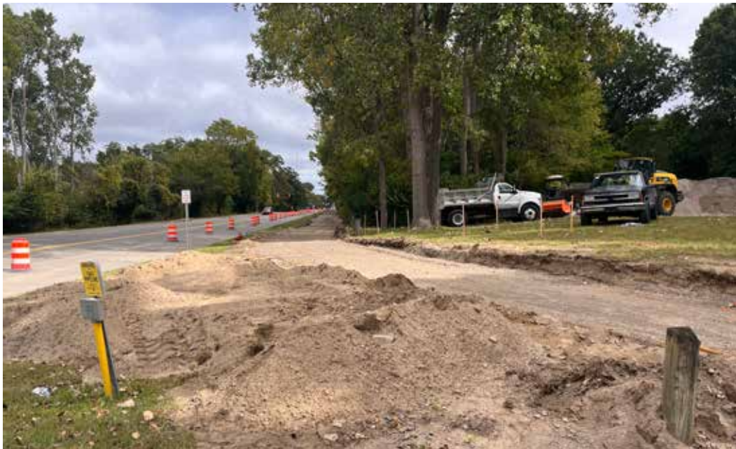
Bauervic Woods path construction.
