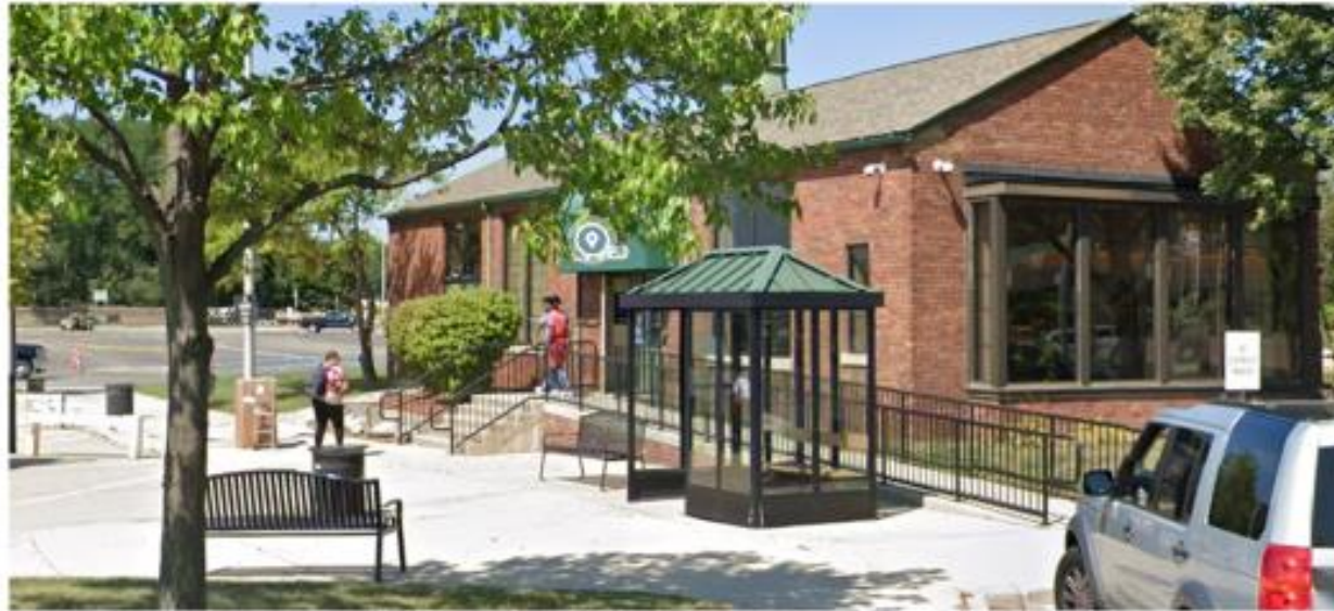
Existing black fixtures at Historic Southfield Transit Center
