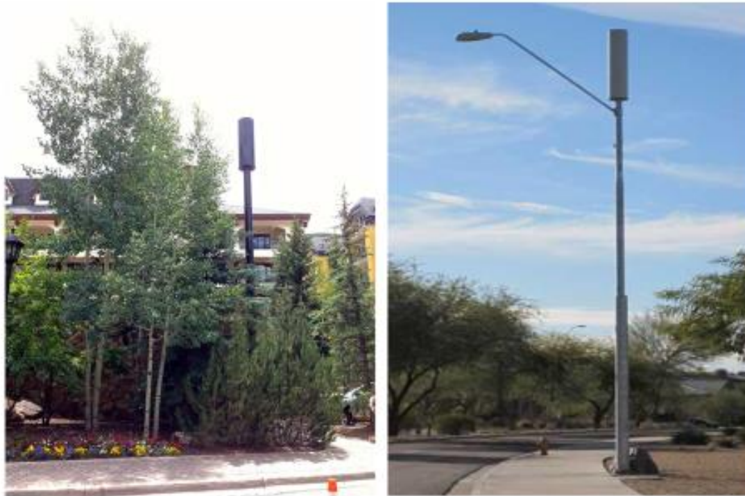
Example small cell wireless facilities - Desirable
