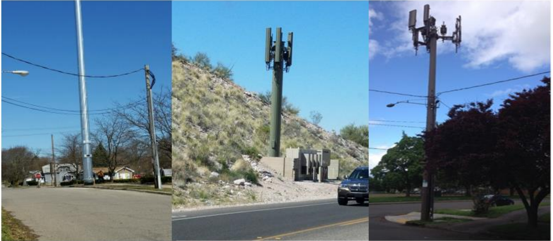
Example large cell wireless facilities – Undesirable
